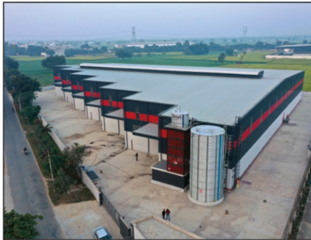
NCR WAREHOUSING PVT. LTD. Location - Gurgaon, Haryana
