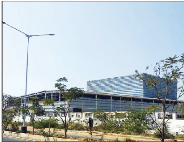
SEPCO ENGINEERING PVT. LTD. Location - Sanand, Gujarat
