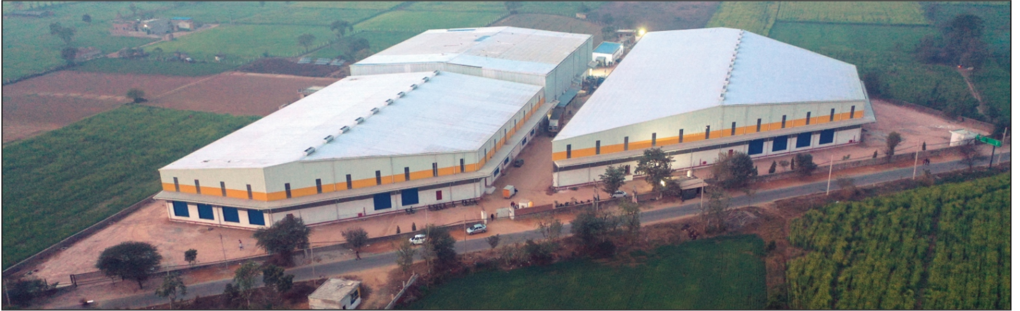
HI-TECH WAREHOUSE PVT. LTD. Location - Gurgaon, Haryana
